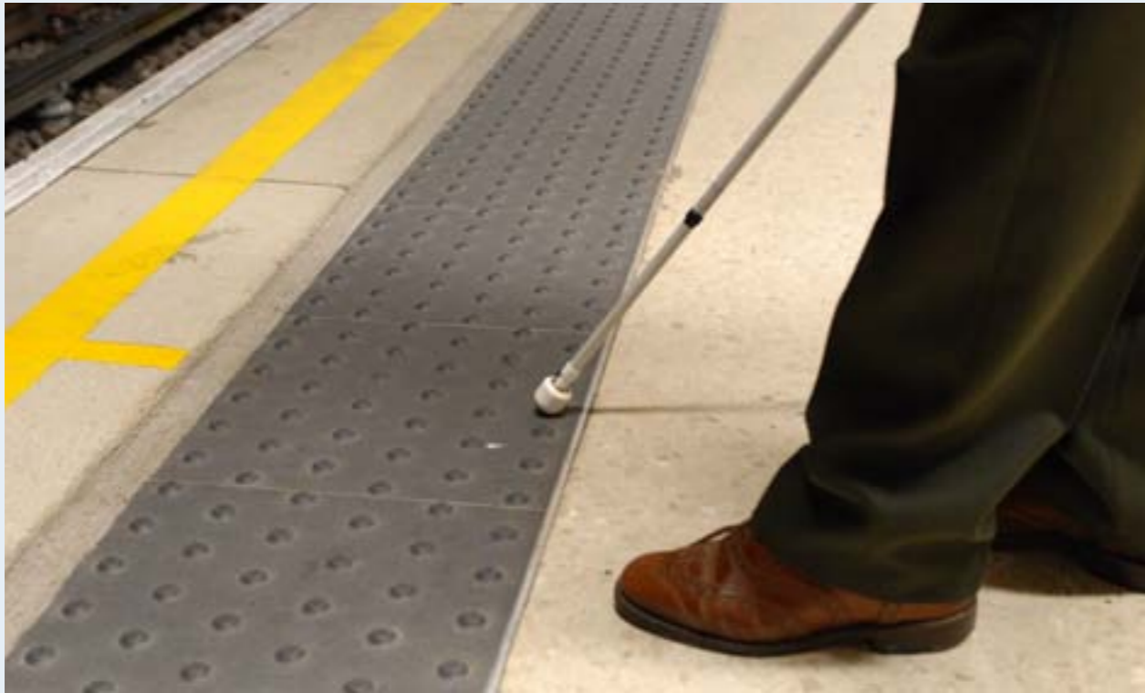
Tactile strips help blind and visually-impaired passengers steer clear of the platform edge
